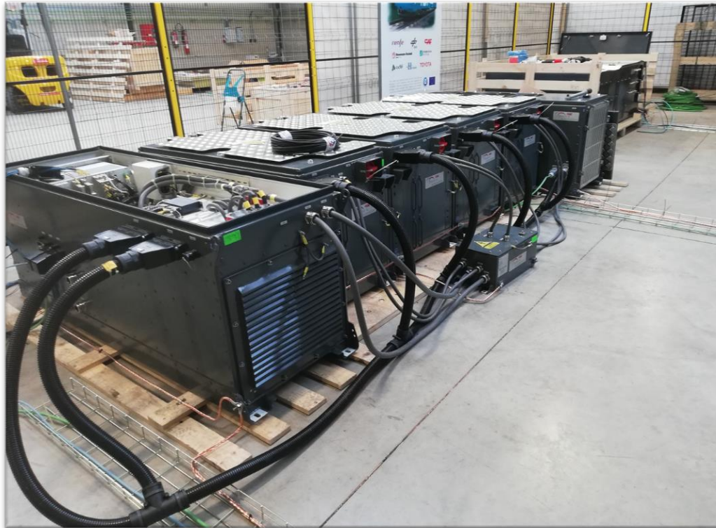
Energy storage with BTMS and DC/DC placing, mechanical and electrical installation
